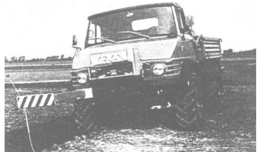
Automatic steering (elektrohydraulic) at ploughing, (BATEL 1968)
